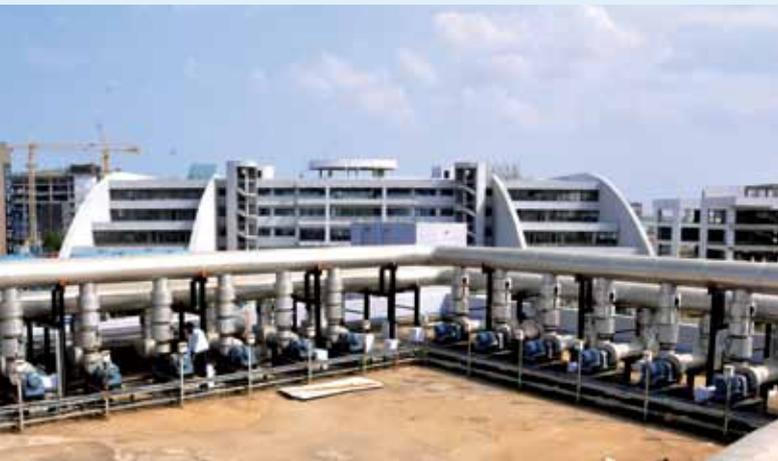
Primary chilled water pumps connected with screw chillers in Phase 1.
