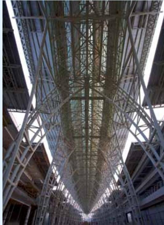
325m long and 45m high, the intricate 8500-ton central spine is designed for relaxation; it was first tested as a bamboo model for stability in strong winds.
