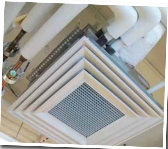
Chilled beam with pipe connection.
