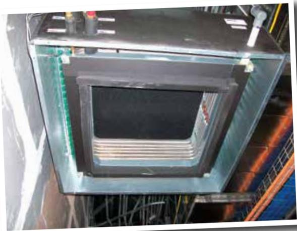
Interior details of chilled beam with coils and nozzles (coloured green).
